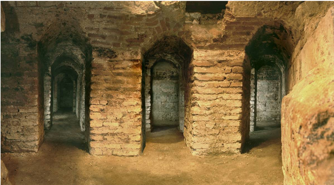
Figure 2: Excavated hypocaust within the bath house located beneath the Cactus House, Nazareth, Israel (Photo: Christine Dalenta)
